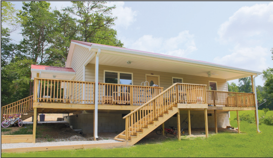
One of the homes built for the Nichols and Fields families by Mountain Outreach in 2015, in its finished form. Facing page: Volunteers and professionals come together to build high-quality, energy-efficient homes for families in need.
